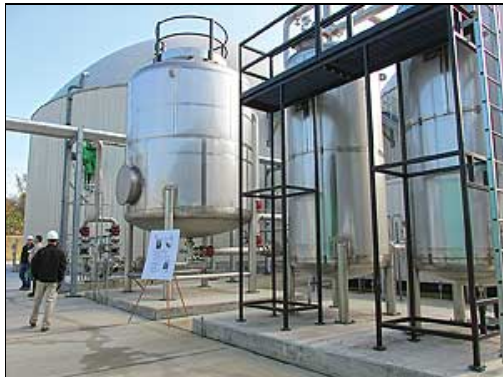
The large tank shown above at left is a digester for biosolids and can hold up to 700,000 gallons, according to KB BioEnergy officials. The smaller tanks hold biosolids before they are digested.
